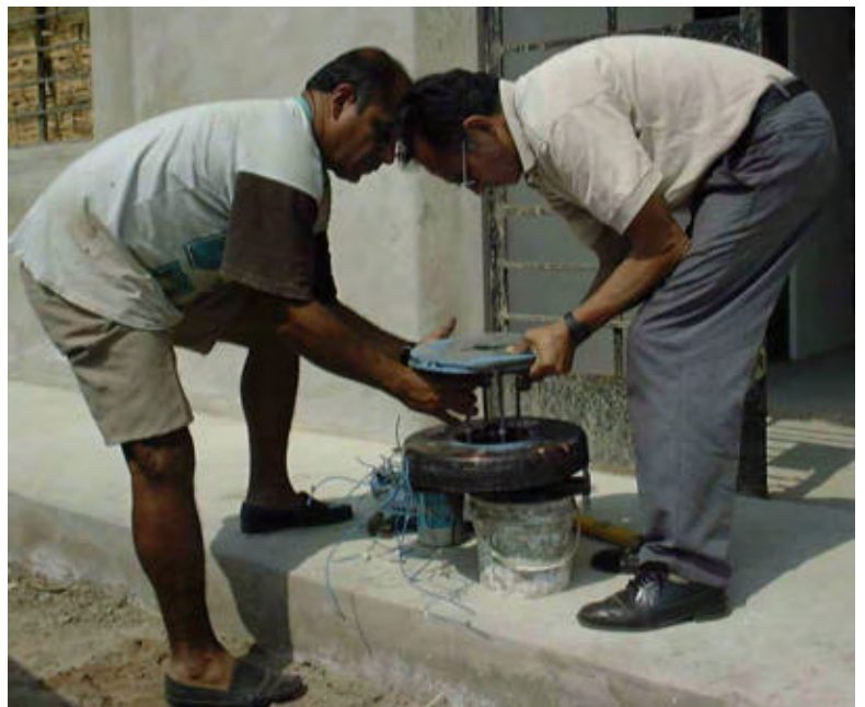
On site assembly in Peru
